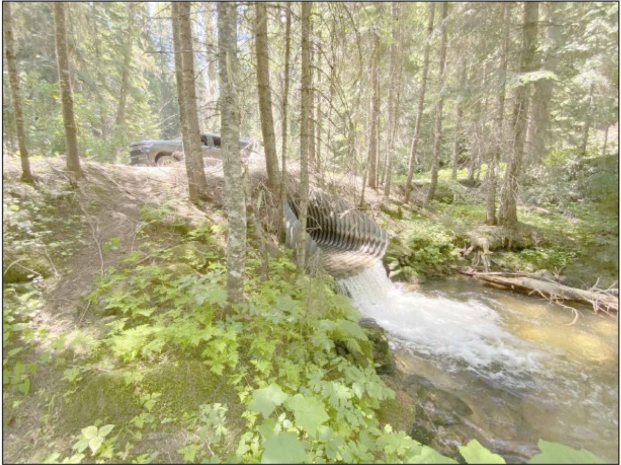
Figure 2. Photo of South Fork Running Creek culvert on USFS road 357.
