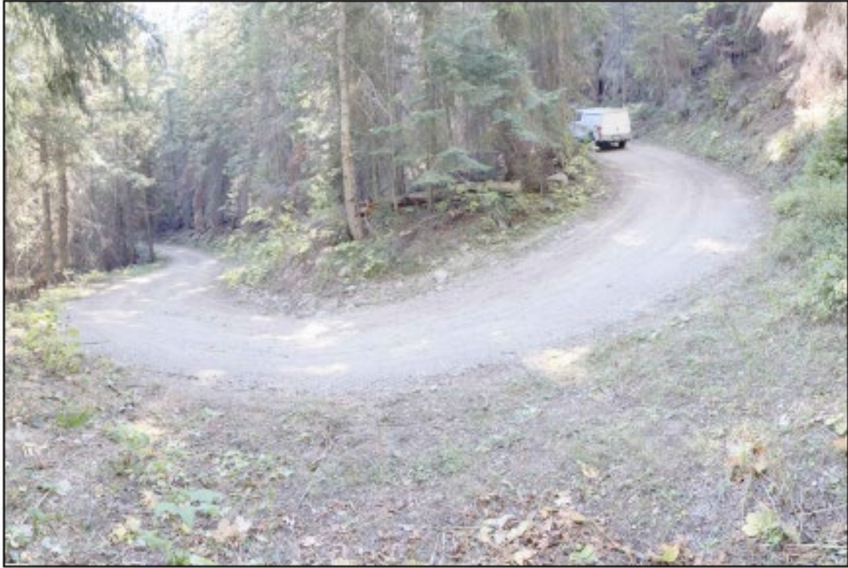
Figure 3. Photo of horseshoe bend #1 on USFS Road 357.
