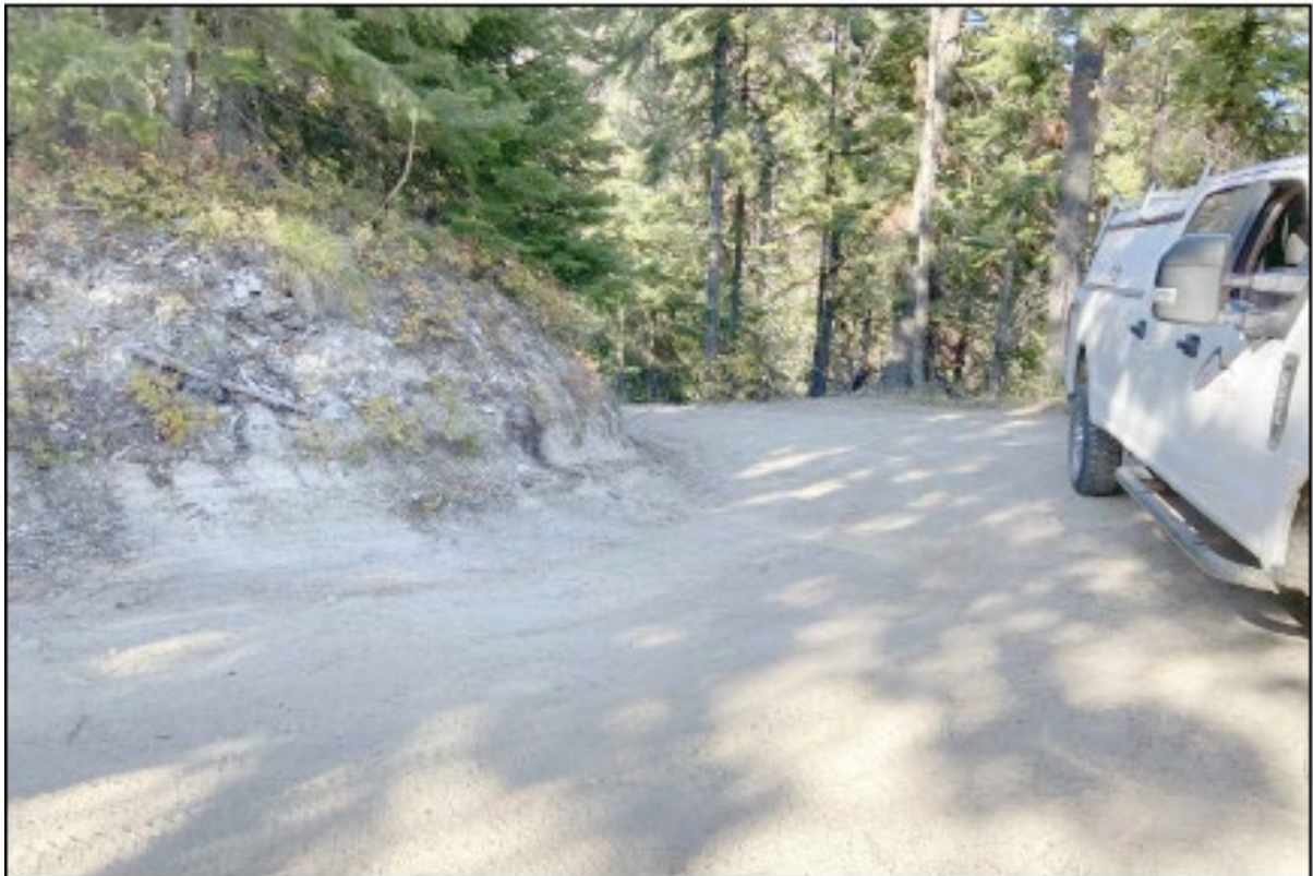
Figure 4. Photo of horseshoe bend #2 on USFS Road 357.
