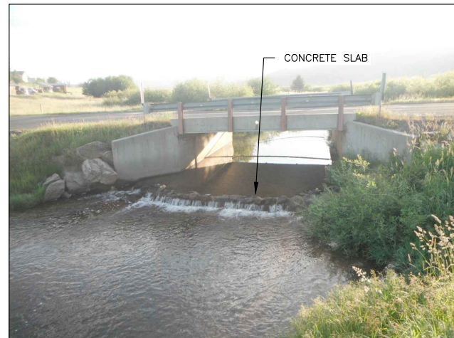
ELEVATION VIEW OF EXISTING BRIDGE LOOKING UPSTREAM (JULY 2014)
