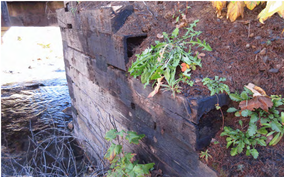
SW wingwall: (CS4) the timber is heavily burnt and is (CS3) leaning 5-degrees.
