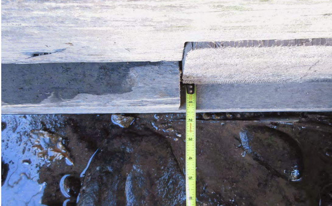
(CS4) North abutment: the bottom timber has a 1.5-inch offset.
