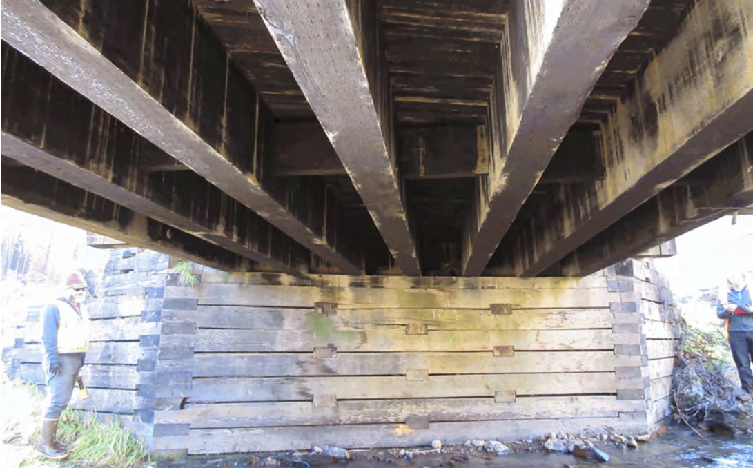
Soffit, superstructure, south abutment, and channel. The abutment has rot and shifting; the top has 1.5-inch settlement.
