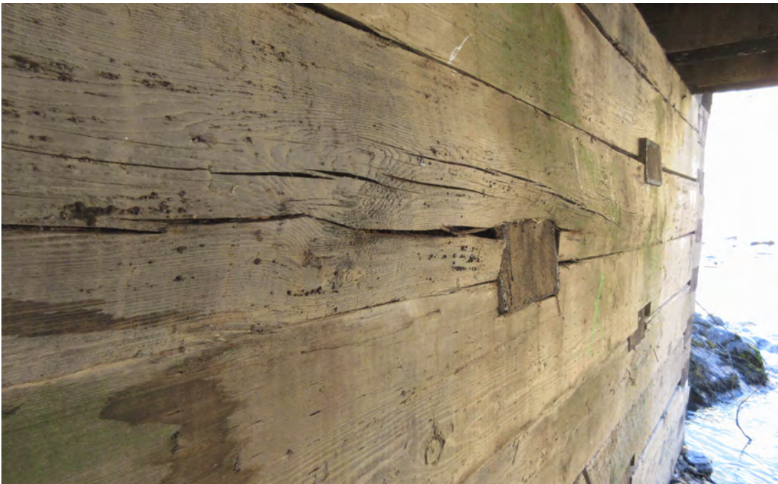
(CS4) South abutment: the third and fourth timbers from the top are fully rotten; the third timber has crushing.
