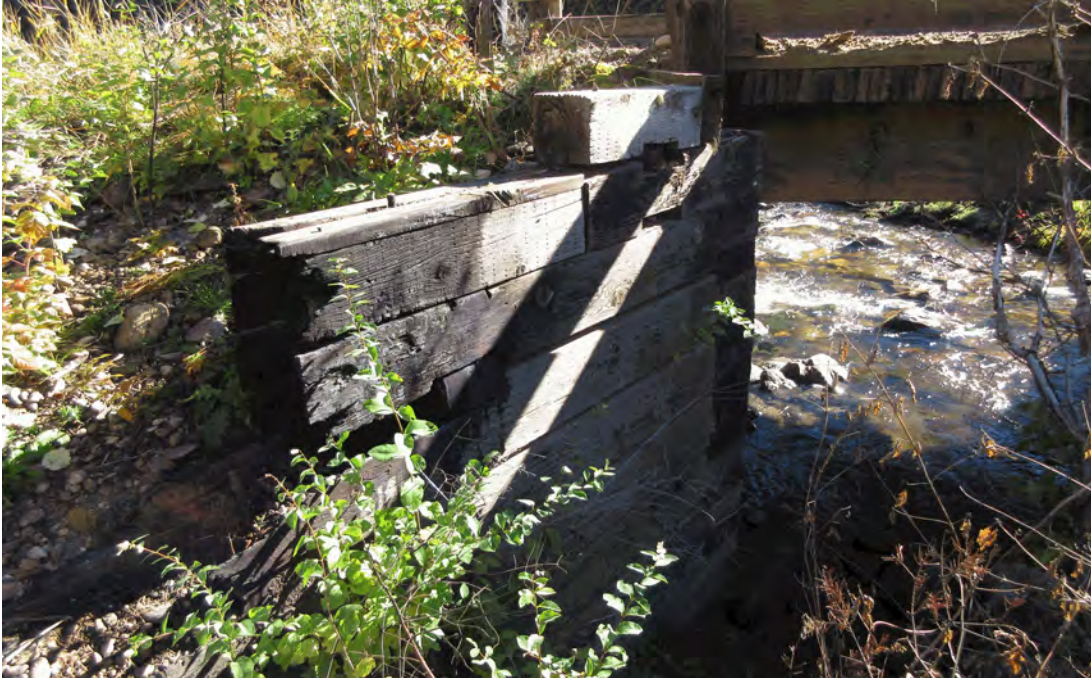
(CS4) NW wingwall: the timber is heavily burnt.
