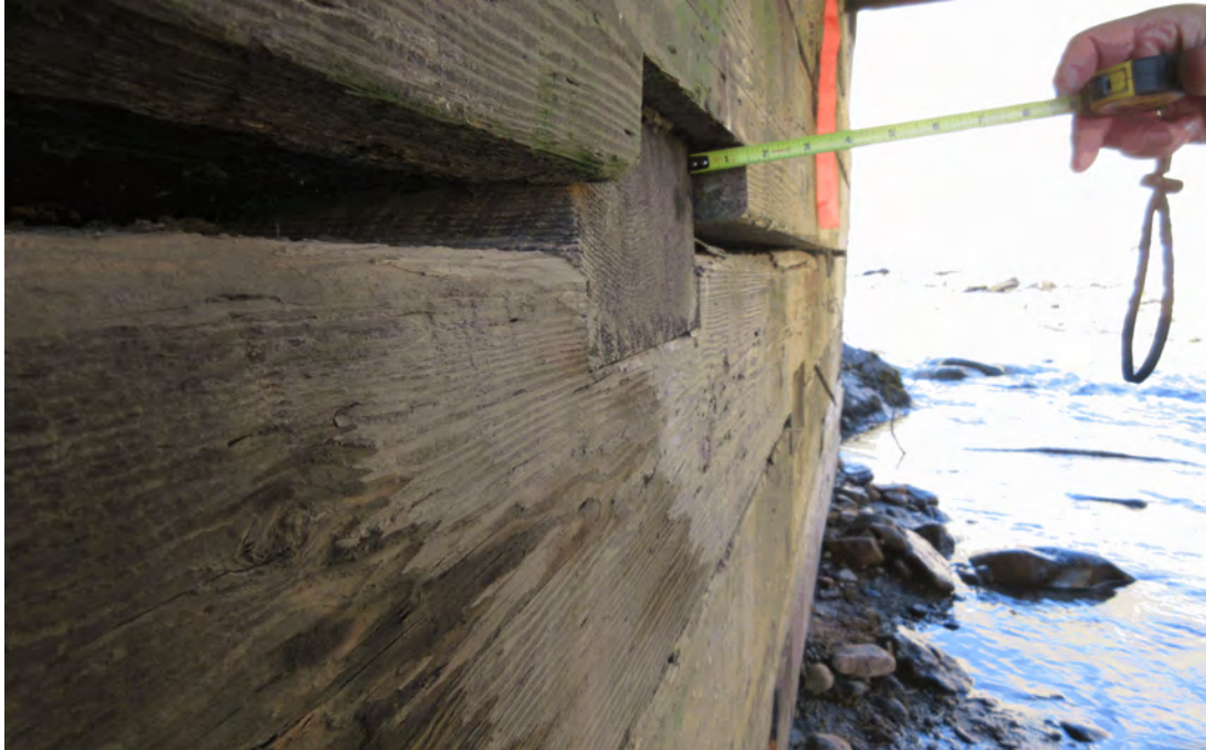
(CS4) South abutment: the 4th beam from the top has a 1.5-inch offset.
