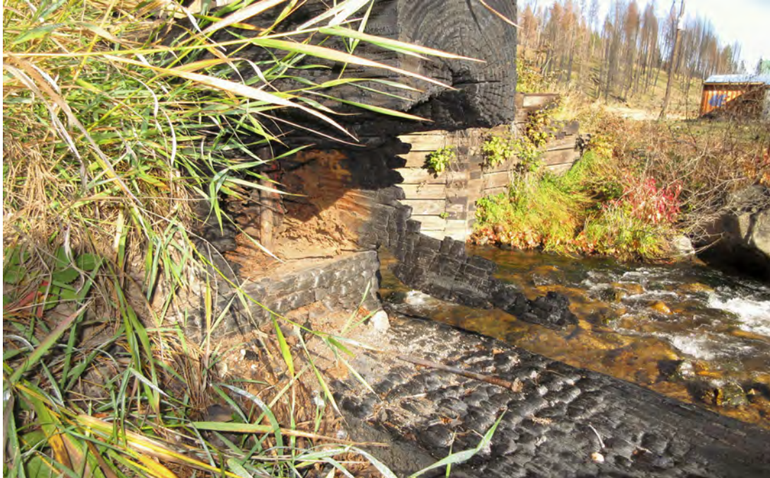
(CS4) SE wingwall: the timber is heavily burnt.
