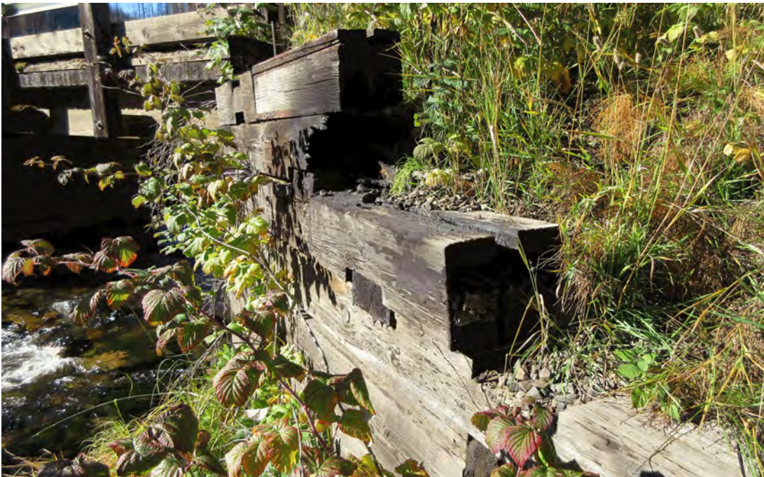
(CS4) NE wingwall: the timber is heavily burnt.
