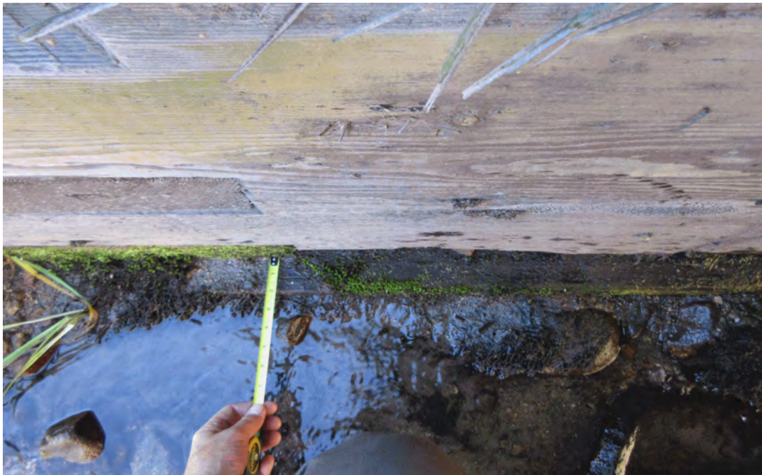
(CS4) South abutment: the bottom timber has a 2-inch offset.
