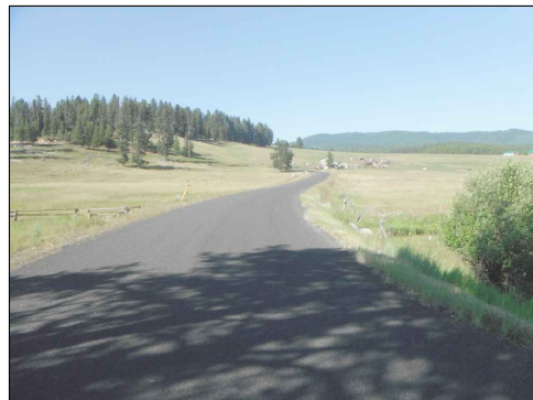
VIEW OF EXISTING APPROACH LOOKING NORTHEAST (JULY 2014)
