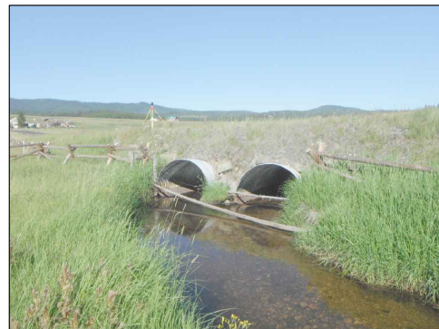
ELEVATION VIEW OF EXISTING CULVERTS LOOKING DOWNSTREAM (JULY 2014)
