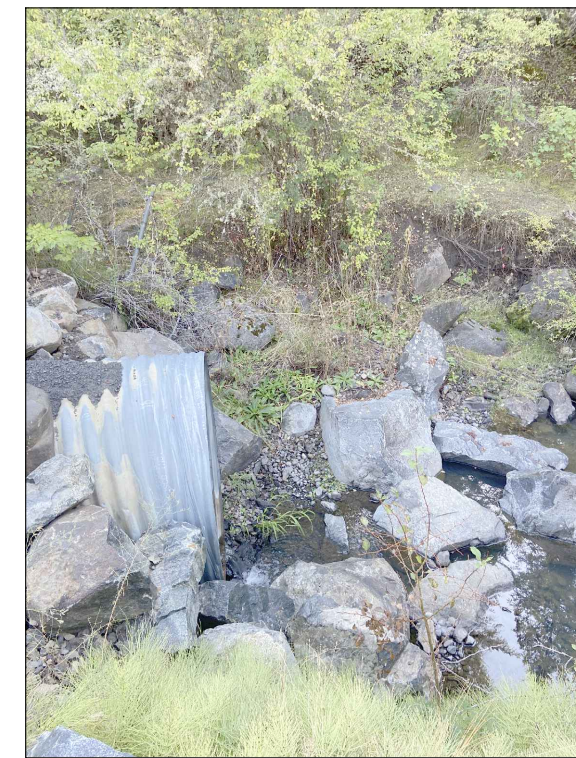
VIEW OF EXISTING CULVERT OUTLET
