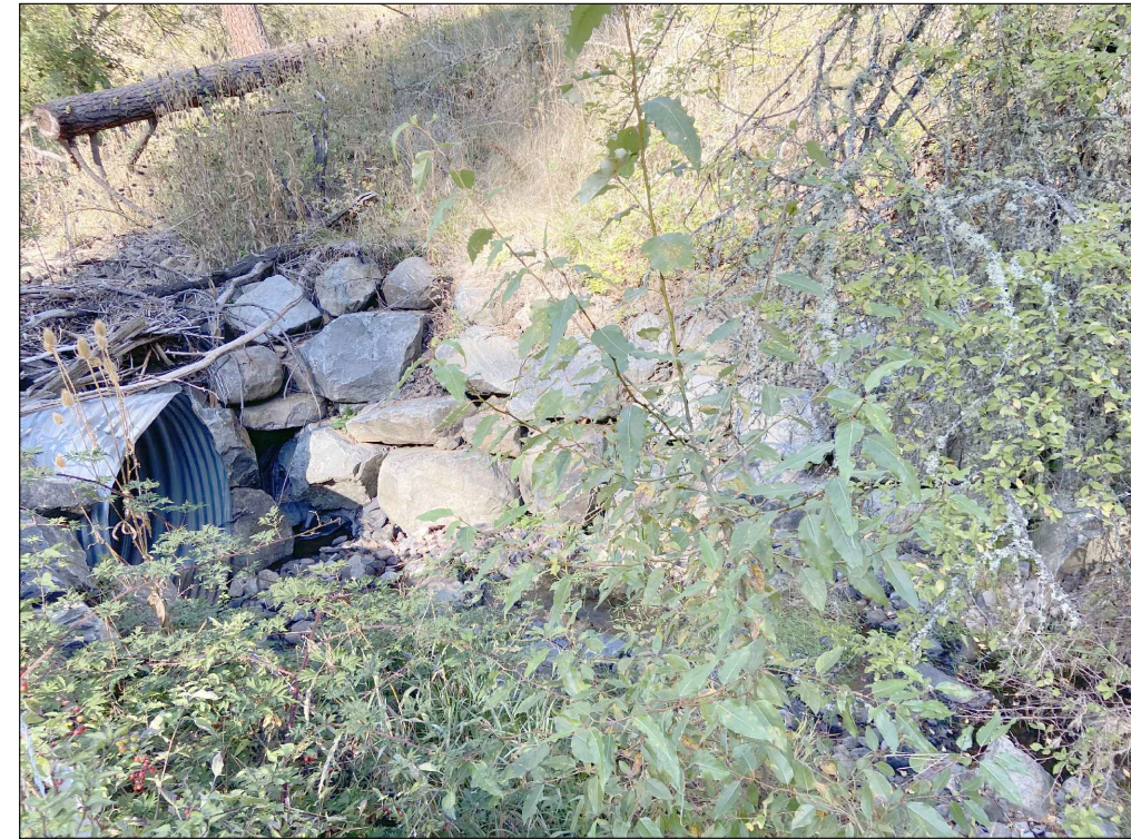
VIEW OF EXISTING CULVERT INLET
