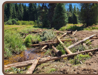
Photo immediately after decommissioning
