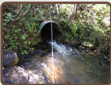
Peter Ready Creek Culvert
