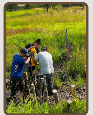
Beaver Dam Construction in Sill Creek
