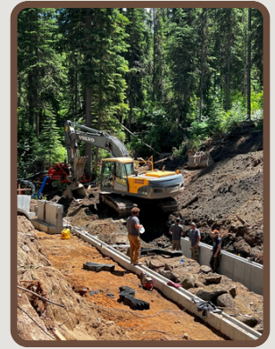
Peter Ready culvert during construction
