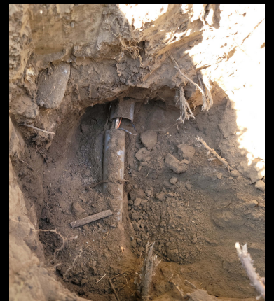
Casino fiber cut we were able to restore.
