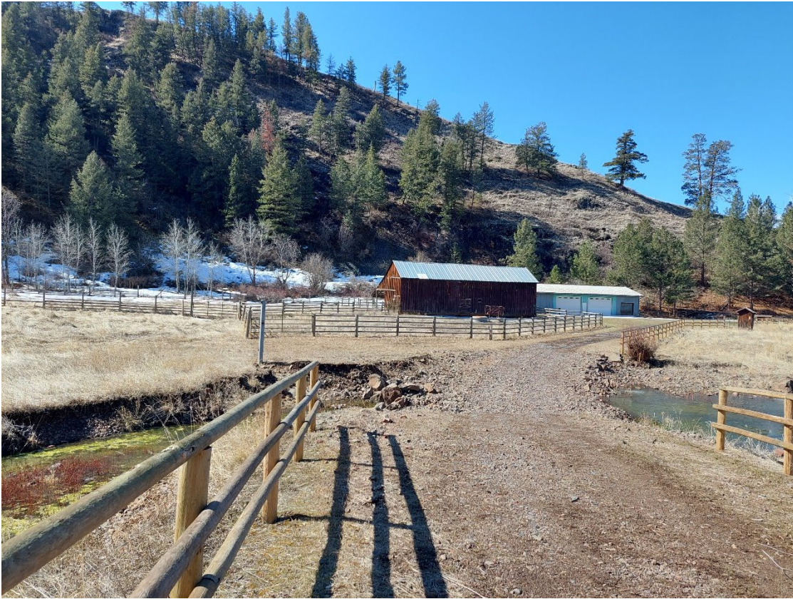
Figure 7. Ford crossing built through the head-cut channel to allow access to the house and other infrastructure on the South side of Chesnimnus Creek.
