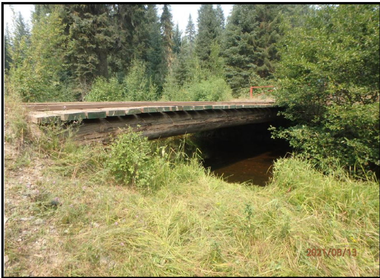
Musselshell Bridge looking Northwest at log girders and wood decking.
