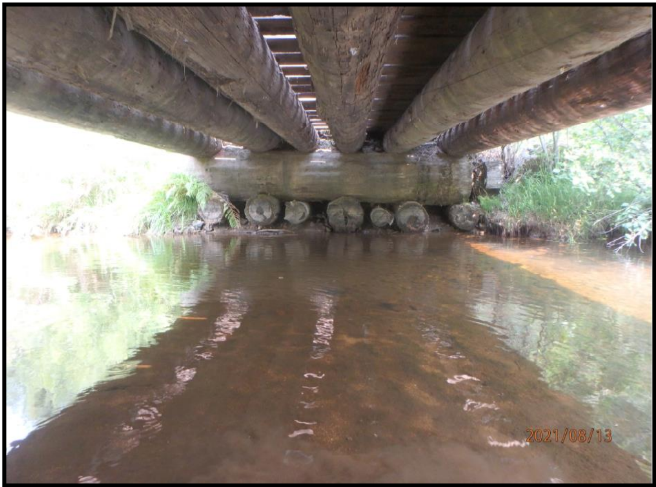
Musselshell bridge looking North at log abutments, supports, and girders.
