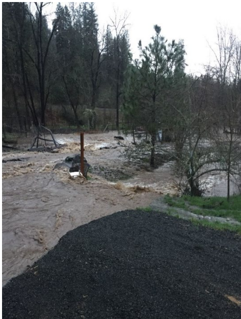
The culvert is undersized and the high flows overtop the driveway, rapidly eroding the streambank, the driveway surface, and the road fill.
