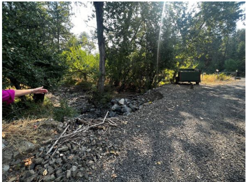
The culvert is undersized and the high flows overtop the driveway, rapidly eroding the streambank, the driveway surface, and the road fill.
