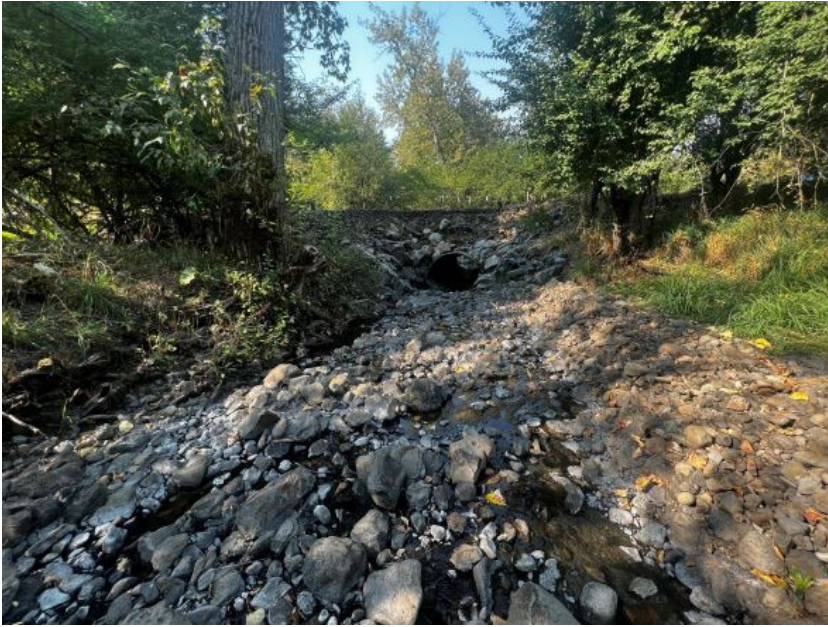
Undersized culvert inlet. The 5.5 ft x 32 ft culvert becomes completely inundated at high flows and tops the driveway in the photo.
