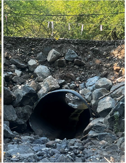
Undersized culvert inlet. The 5.5 ft x 32 ft culvert becomes completely inundated at high flows and tops the driveway in the photo.
