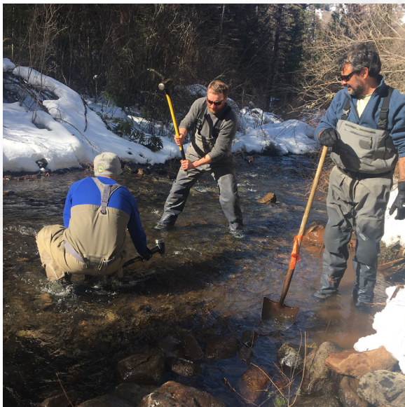
Installing the new 2022 Crazyman Creek weir for adult steelhead monitoring.
