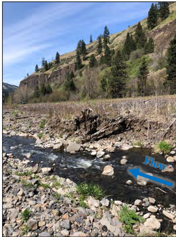
Photograph 6. Existing downcutting within Lapwai Creek. Previously constructed large woody material now perched.
