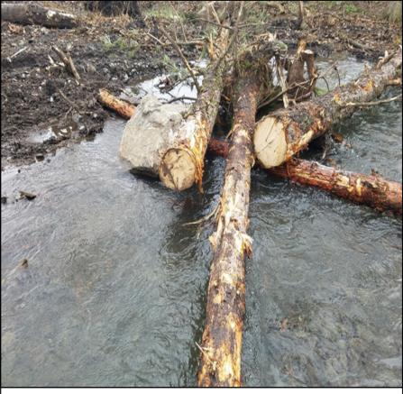
Sweetwater Creek fully diverted into new channel with habitat structure
